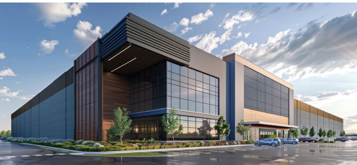
Developer adding $185M campus to New Albany data center boom
